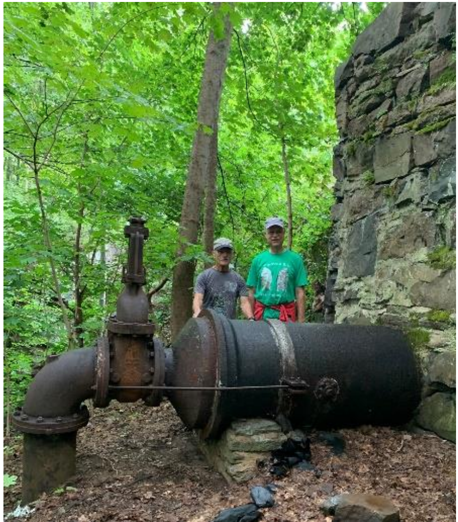
Penstock and valve controlled outflow from dam
